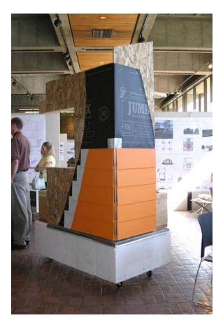
Figure 7: Students Ryan Berry and Adam Naylor construct a prototype corner of their design proposal which implements Insulated Concrete Foundation (ICF), panelized walls utilizing 2 x 6 @ 24" o.c. efficient framing, and cement board siding.
